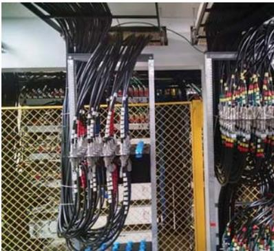
409 antennas and 86 remote equipment dual-node locations. This equipment also required a head-end equipment room, comprising 1,400 square feet with 3x10 ton HVAC units and 400 amp, three-phase power.
